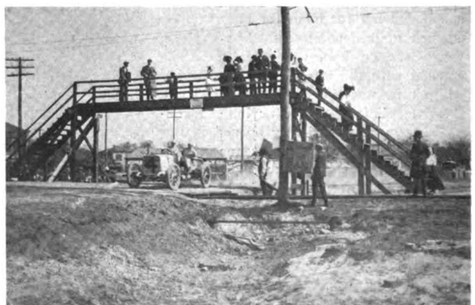
In Two Places the Road Was Bridged.
